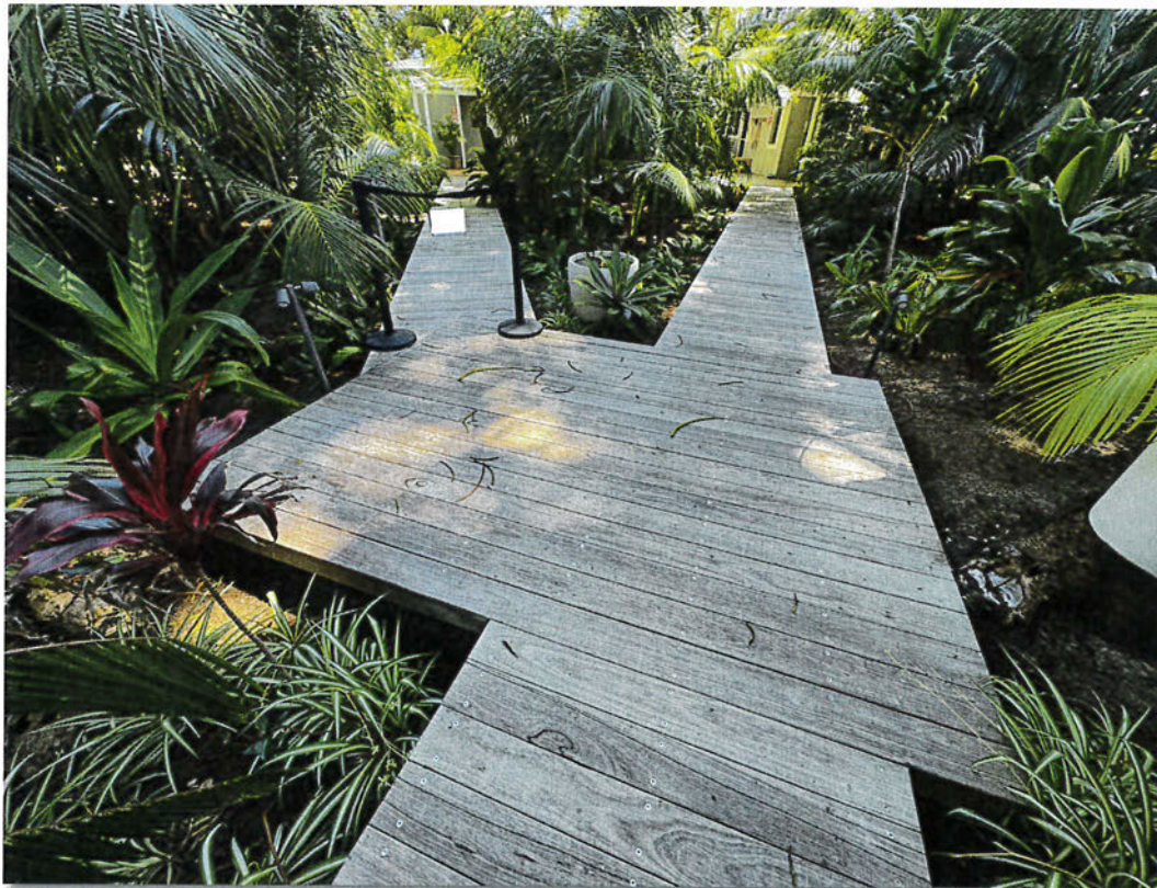
Figure 6 - Raised timber boardwalk access to existing building (left boardwalk)
