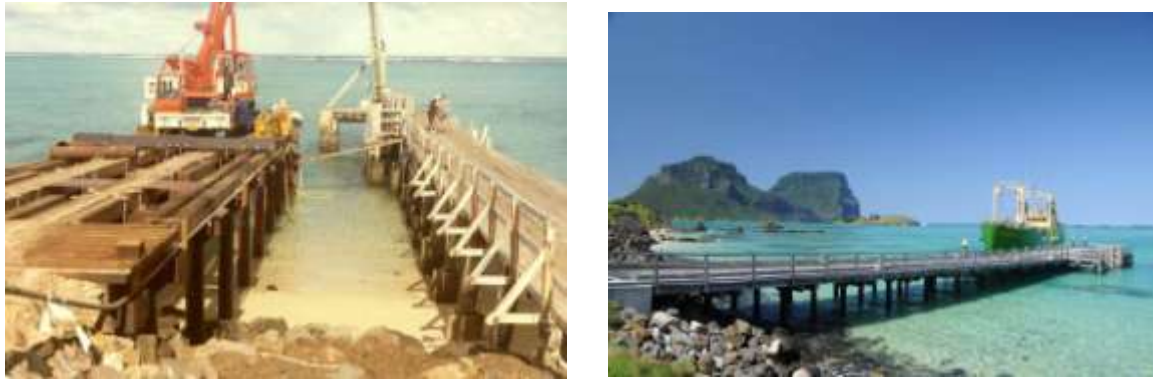
Figure 154 (Left): The new jetty under construction, with the old jetty with hoist beside it. (Photo: Miscellaneous prints 4, Mis4-153, LHI Museum Collection); (right): The new jetty with MV Island Trader docked. (Photo: Chris Betteridge, 1 March 2009).
