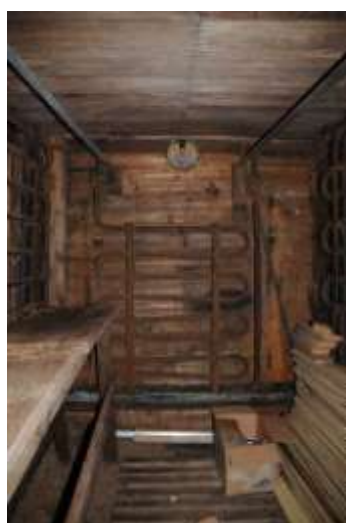
Figure 20 The cool room in a building at the rear of 'Thornleigh', the Dignam residence in Lagoon Road retains relatively intact evidence of past refrigeration technology. (Photo: Chris Betteridge, 21 March 2010)
