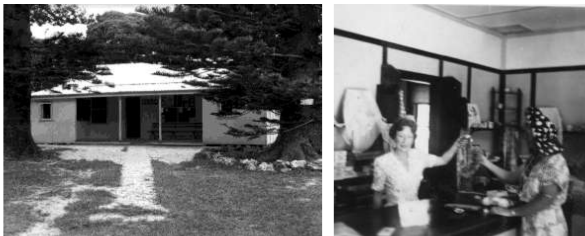
Figure 19 (Left) Undated photograph of Thompson's Store. The Norfolk Island Pine trees have gone. The store survives in a much altered state, and with major issues arising from the deteriorating asbestos cement cladding. (Photo: Miscellaneous Prints Mis4-148, LHI Museum Collection); (Right): Undated photo of Babe Green (née Payten) serving a customer in The Gift Store (Photo: Babe Payten Prints 1927-60, BP50, LHI Museum Collection).
