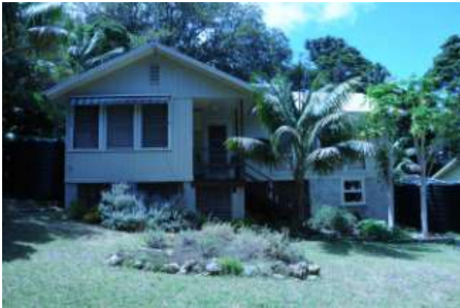
Figure 219 One of the prefabricated houses erected on Lord Howe Island for the Department of Civil Aviation. (Photo: Chris Betteridge, 3 December 2009)
