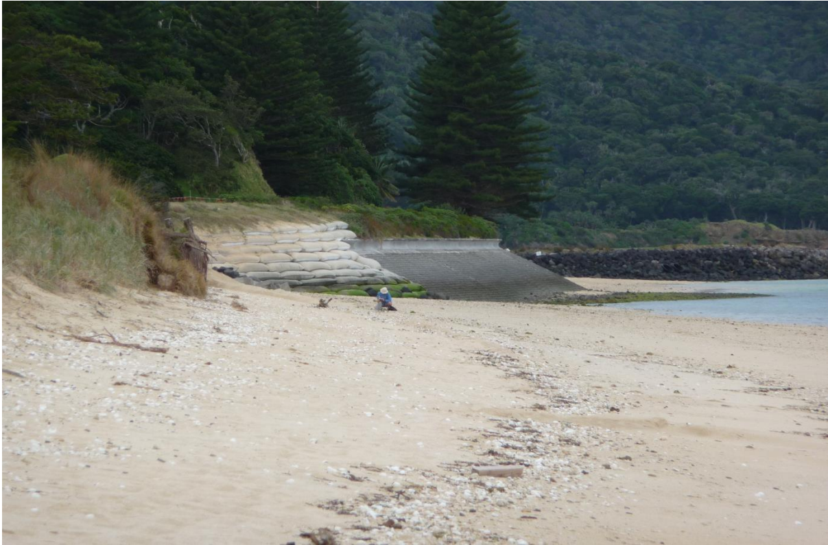
Figure 6: View of sand-filled geotextile container wall, Seabee revetment and runway revetment from the southern end of Lagoon Beach, 28 August 2012
