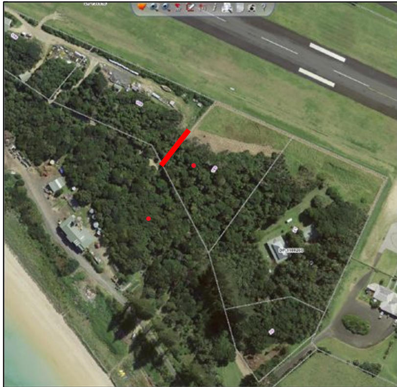
Figure B: Approximate location of the existing track running along the boundary of lot 183 and lot 109
