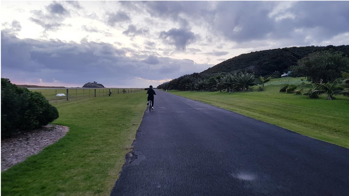
Plate 7 – Looking north-west from Lagoon Road adjacent to the airstrip towards the Lagoon. If the proposed runway extension were to progress further, this portion of the road would need a new realignment in order to avoid vehicles and the fence line impinging the ‘fly-over area plane’ and OLS restrictions.
