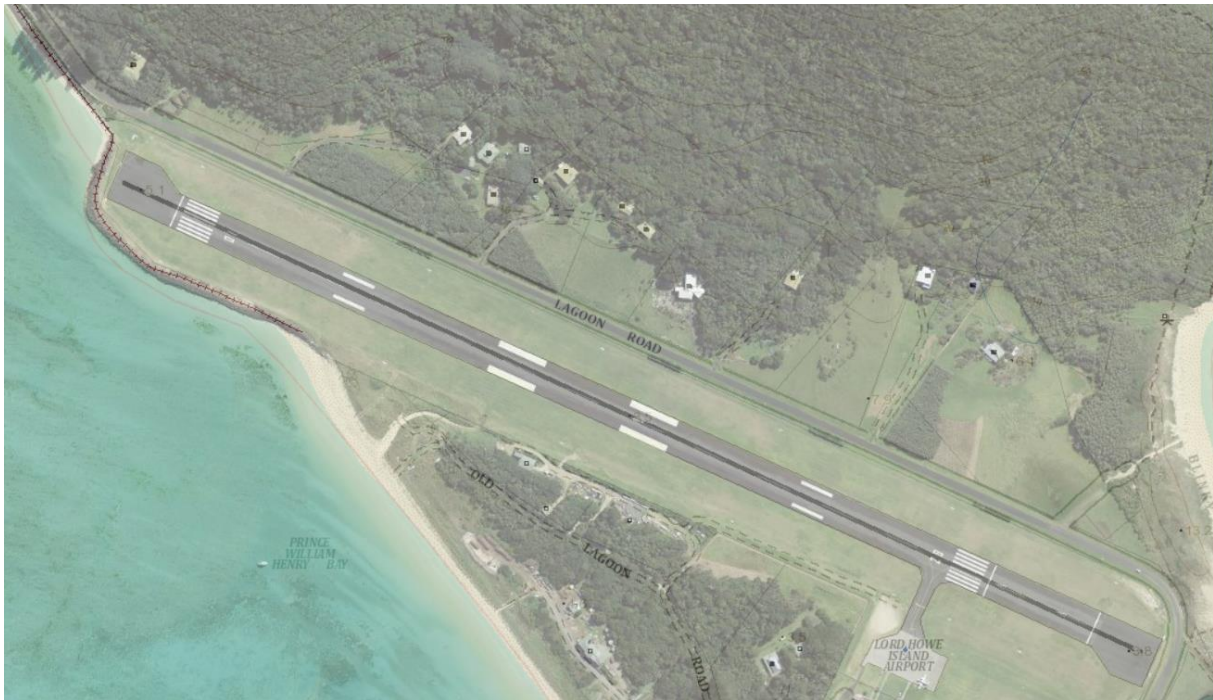
Figure 3-5 Lagoon Road adjacent to the airstrip (SIX Maps)
