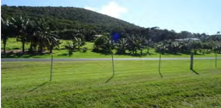
Figure 29 Existing perimeter security fence
