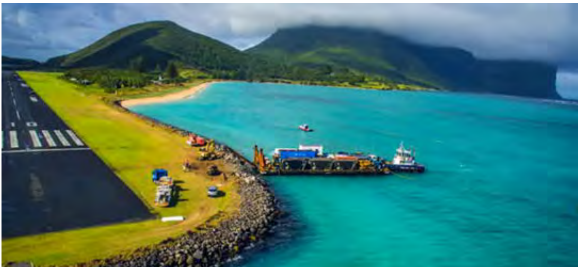
Figure 13 Plant and material delivery for the 2014 runway overlay project
