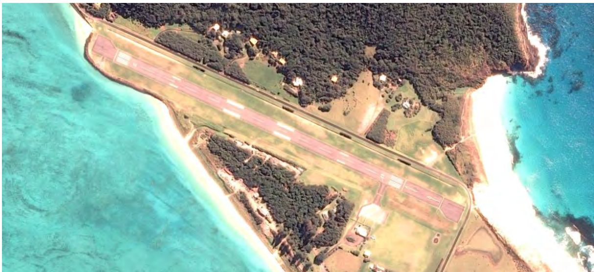
Figure 1-1 Aerial photo of the existing airport layout
