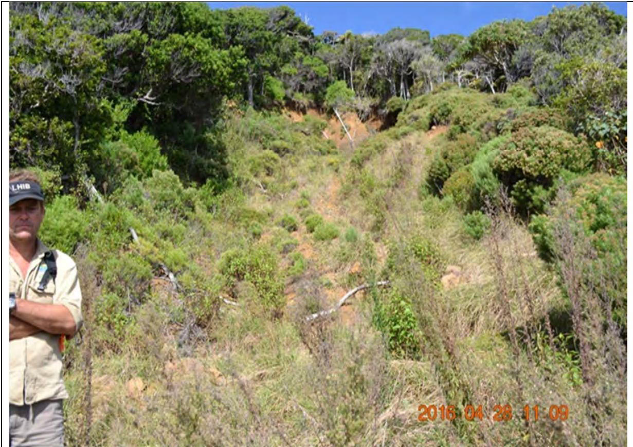
Site 5 Lower mid slope area of slide looking upslope to the south west towards backs scarp
