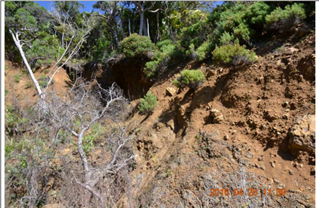
Site 7 Mid to upper slope area looking south west to exposed colluvial batters with rock "floaters" that could detach down slope towards the track
