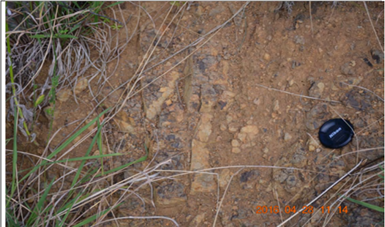
Site 6-exposed floor of mid-slope section of slide showing weathered outcrop of weathered but competent Boat Harbour Breccia bedrock
