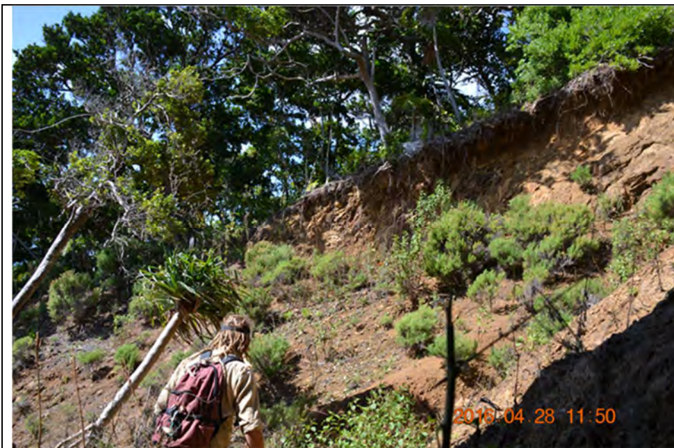
Site 8 Backscarp area looking toward the south eastern colluvial batters
