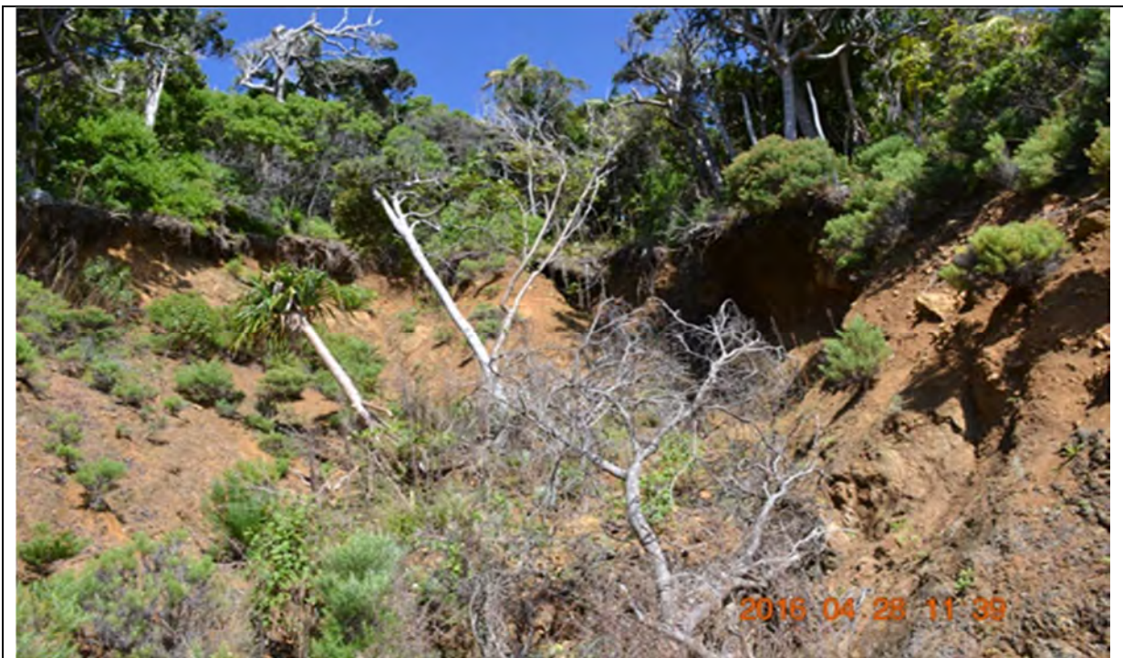
Site 7 Mid to upper slope area looking south west towards backscarp area
