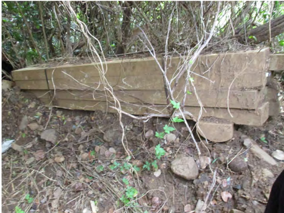
Photo 8- Timber beams and debris washed down slope by possibly 25m from proposed construction site to the lower walking track section to the north west.
