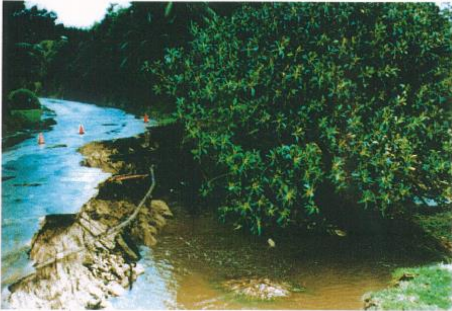
Photograph 17: Road Damage at Cobbys Corner caused by flood overflow
