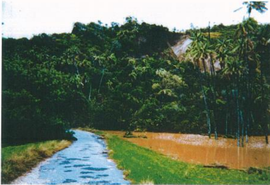
Photograph 19: Major land slip closing road south of Kings Beach
