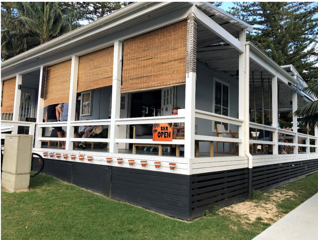
Figure 3: Front corner of development as constructed
