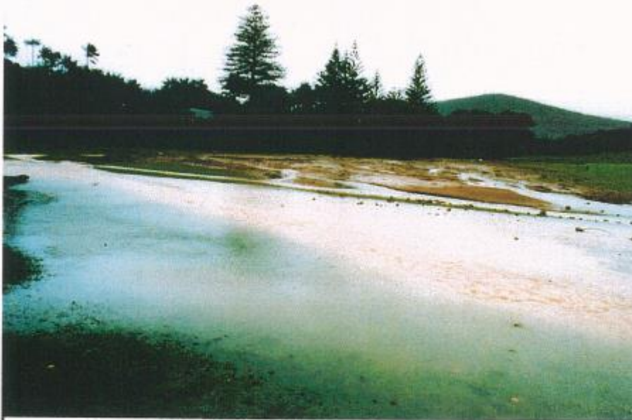
Photograph 18: Silt deposition on Golf Course upstream of Ms Wilson's house
