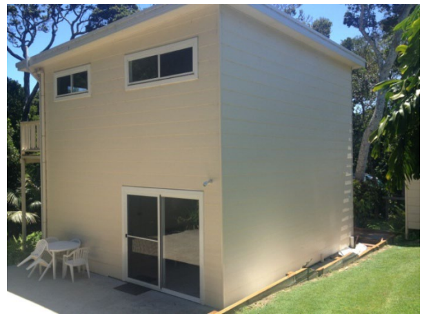
Figure 7 Infrastructure building that is the subject of this application
