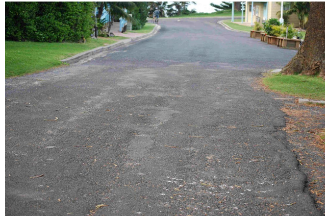
Ned's Beach Road – the highest trafficked location.
