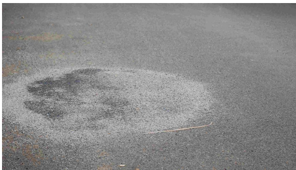
Typical patch using cold bitumen and 7mm gravel.
