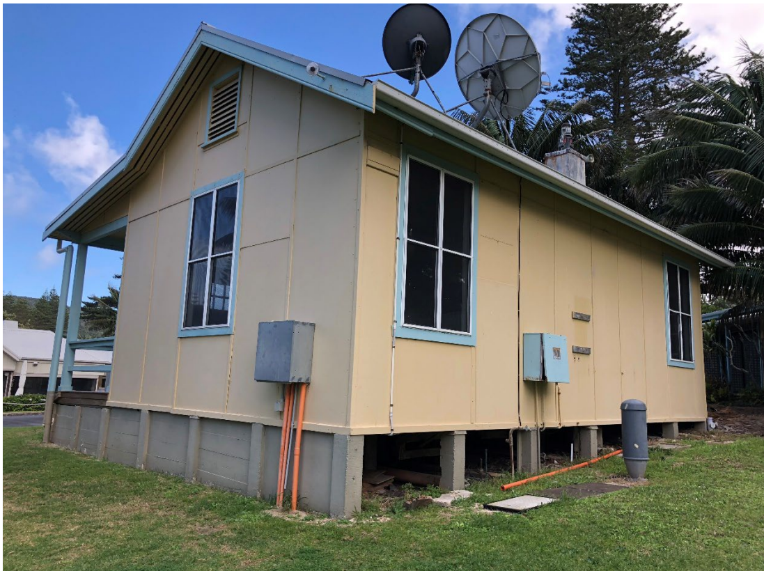
Figure 2: Western (side) & southern (rear) elevations of existing building.
