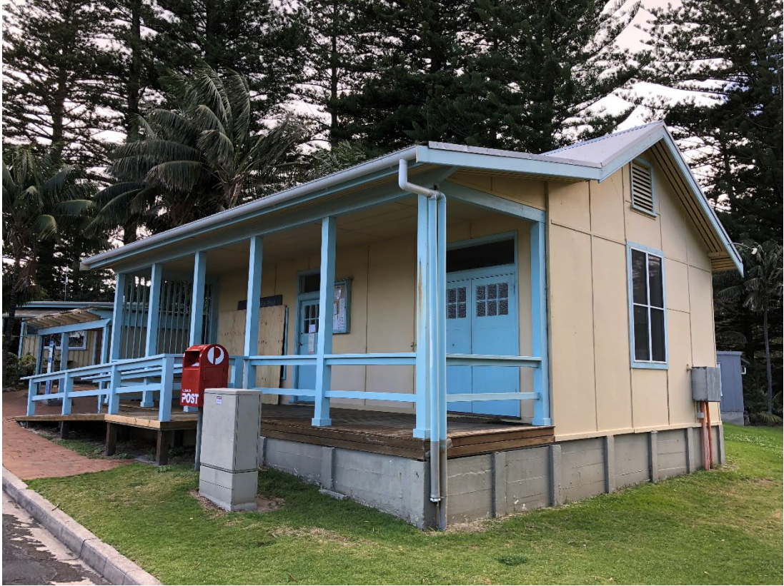
Figure 1: Northern (front-to Ned's Beach Road) & western (side) elevations of existing building.
