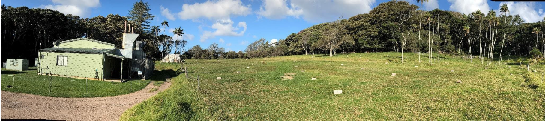
Figure 2: LHI Powerhouse & Location of Proposed Battery Storage and Eastern Component of Solar Array Area
