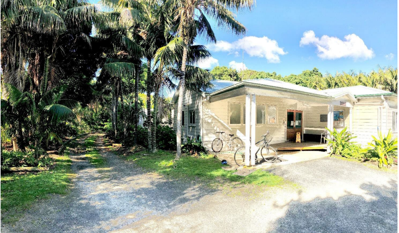
Figure 4: Front of existing LHI Hospital, side driveway & location of proposed attached ambulance garage
