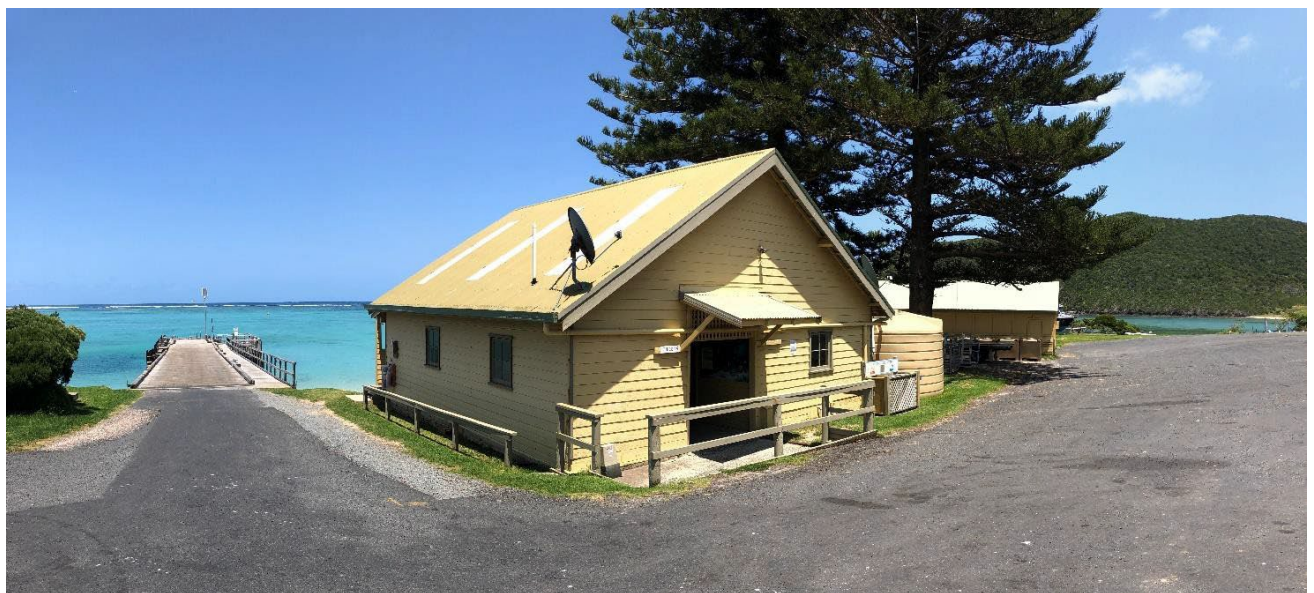
Figure 2: LHI Wharf & Cargo Shed/ Radio Shack to south east of proposed Marine Rescue facility
