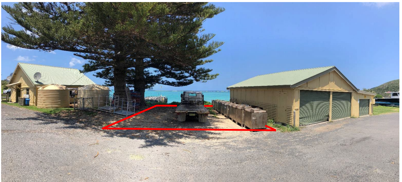
Figure 6: Left to Right: Existing LHI Cargo Shed/ 'Radio Shack', proposed Marine Rescue Operations site (approx. highlighted) & Combined LHI, RMS, Marine Park office, storage & annex
