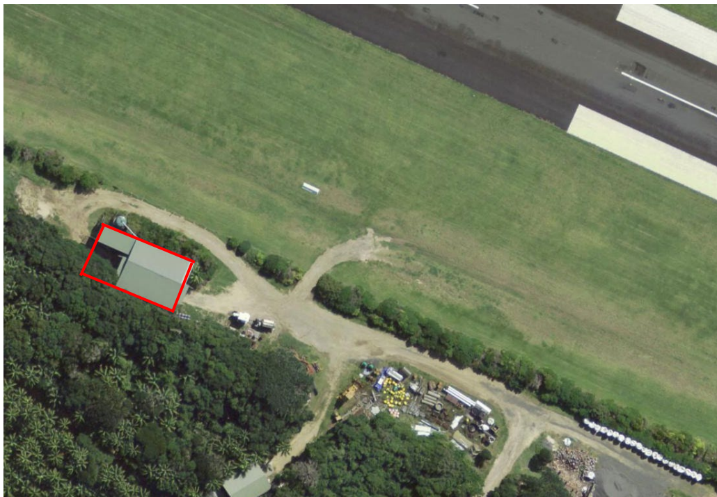
Figure 1 – Existing building to be demolished and removed. Source: Six Maps
