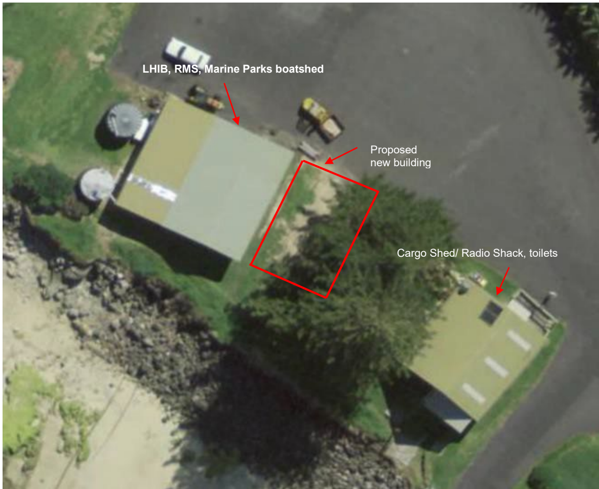
Figure 5: Aerial View of the existing boatshed buildings & proposed site of new Marine Rescue NSW building. Source: Six Maps
