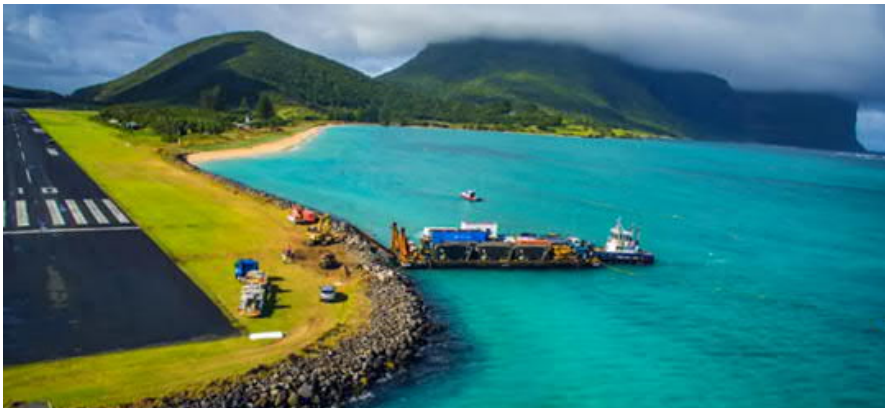
Figure 9 Plant and material delivery for the 2014 runway overlay project
