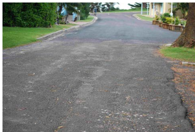
Ned's Beach Road – the highest trafficked location.
