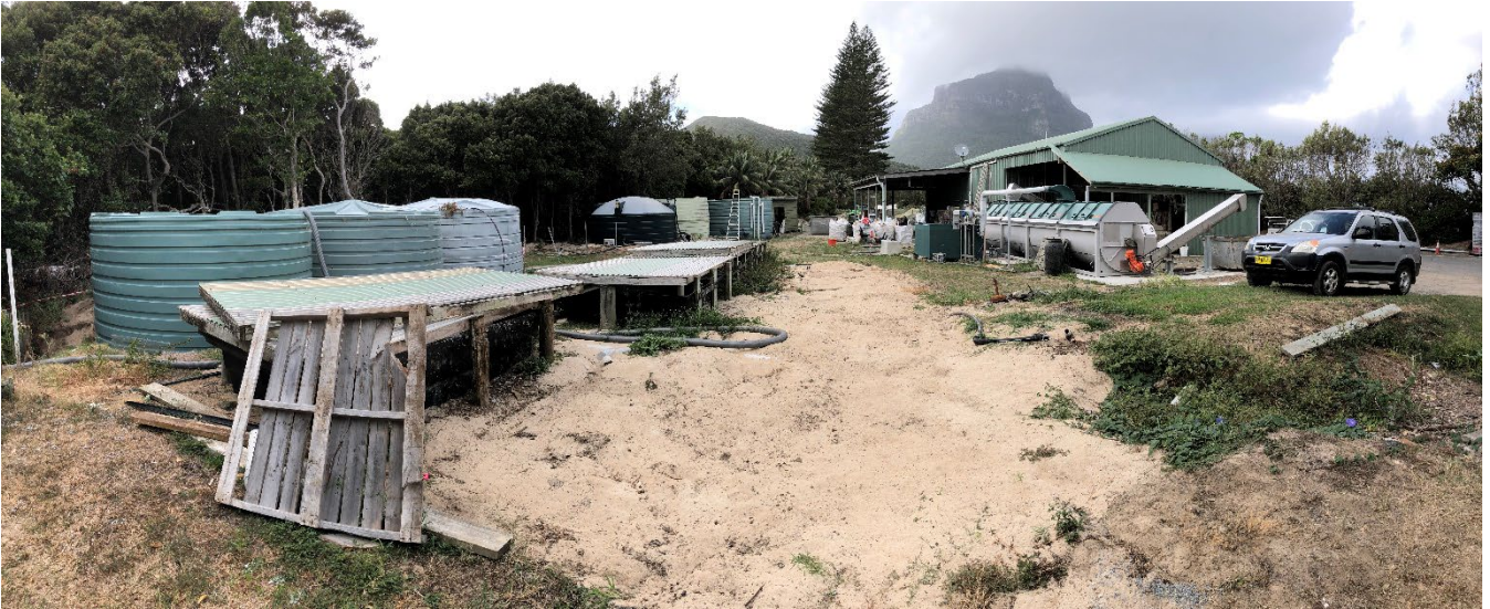
Figure 4: Existing Sludge Drying Beds and Location of Proposed Sludge Dewatering System at the LHIB WMF
