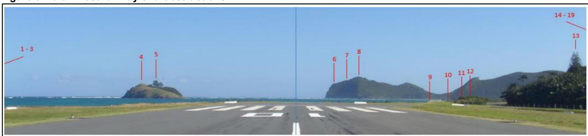
Figure 9 North West runway end obstructions
