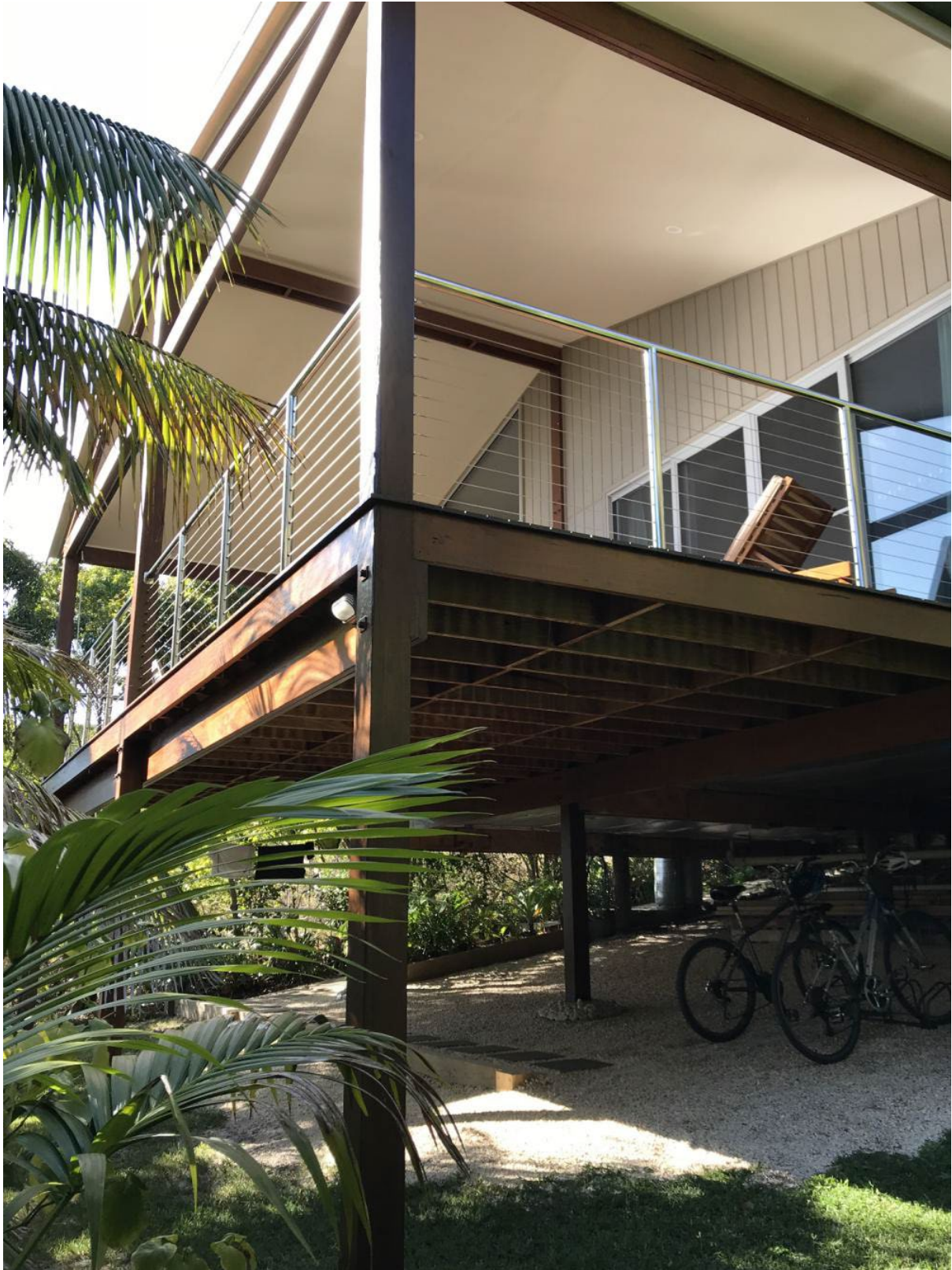
Above: Existing elevated west facing deck of the Treehouse tourist accommodation unit on Portion 295
