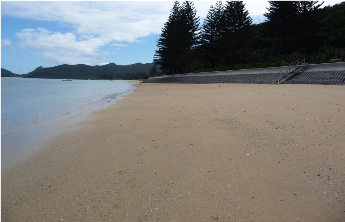
Figure A2: Looking north along Seabee wall at southern end of Lagoon Beach
