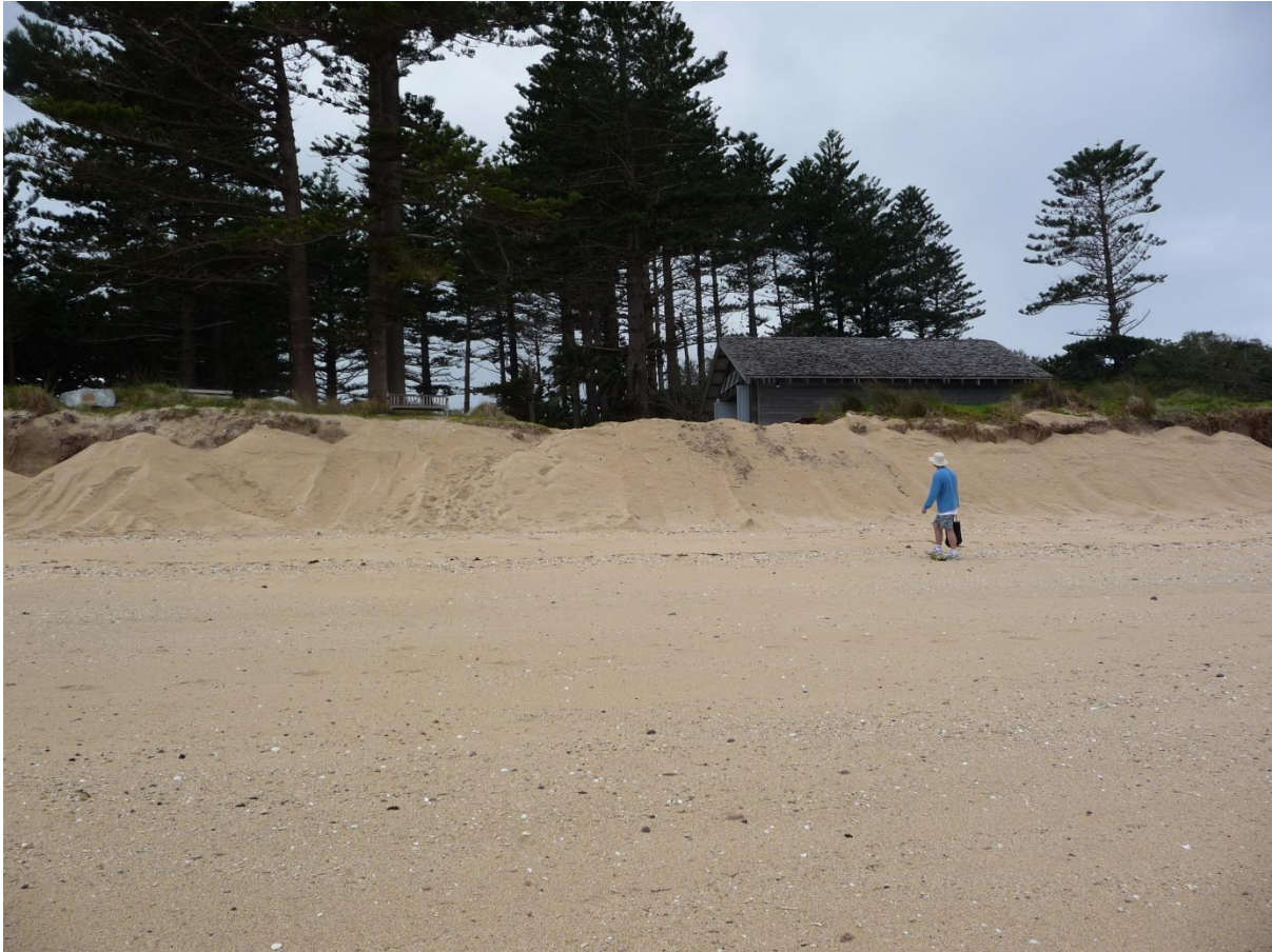
Figure 31: Sand from beach scraping pushed against erosion escarpment at Pinetrees boatshed, 28 August 2012
