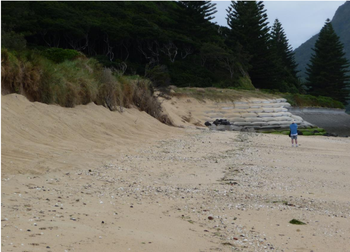
Figure A4: Sand-filled geotextile containers north of Seabee wall at Lagoon Beach
