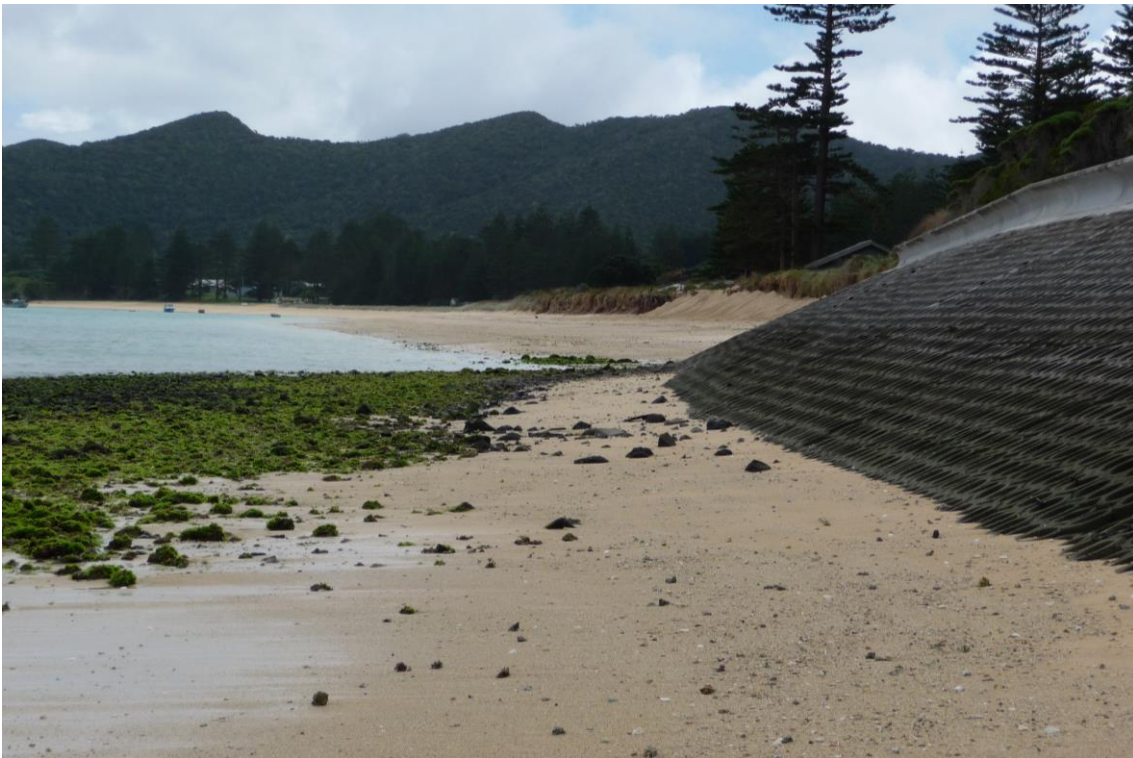
Figure A3: Northern end of Seabee wall at Lagoon Beach, looking north
