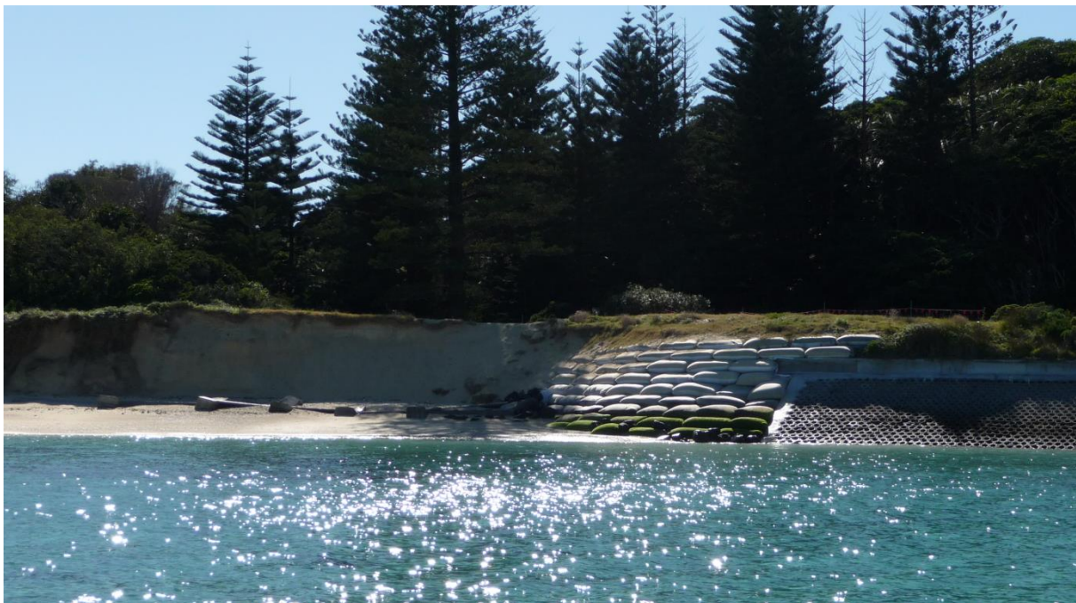
Figure 7: View (left to right) of eroding dune with concrete and rock on beach, sand-filled geotextile container wall and Seabee revetment (29 August 2012)
