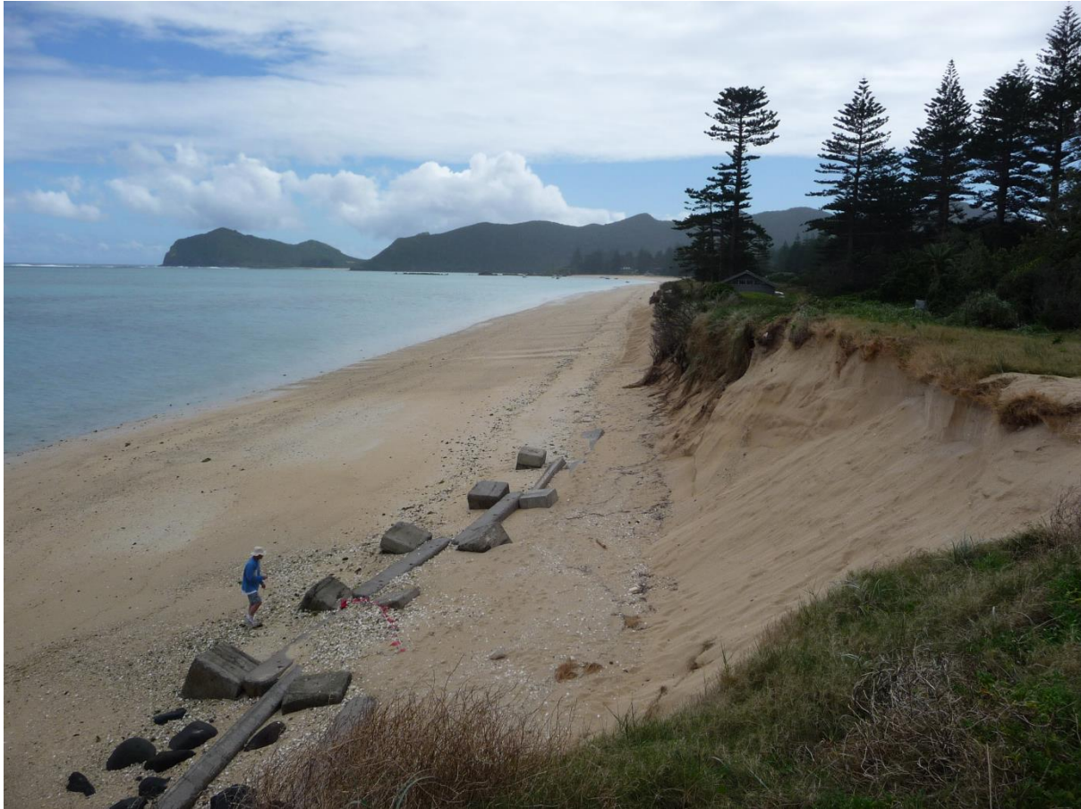
Figure 5: Concrete north of sand-filled geotextile container wall, 28 August 2012
