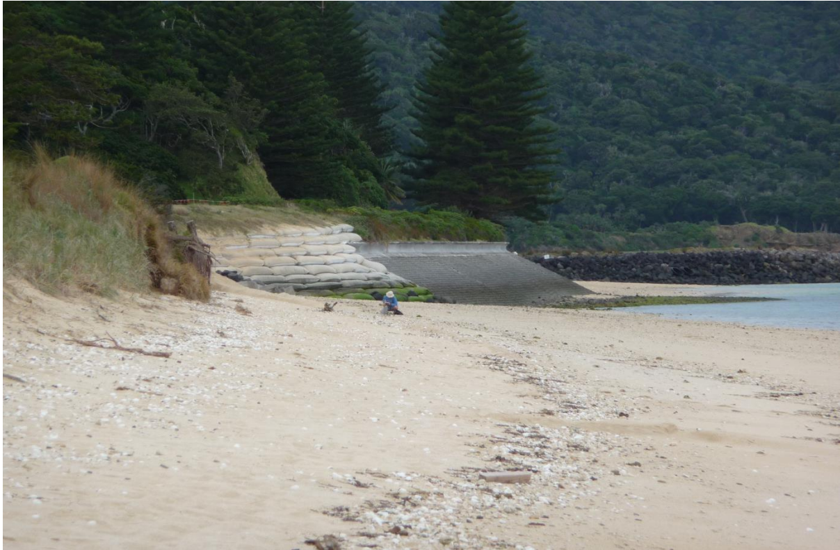
Figure 6: View of sand-filled geotextile container wall, Seabee revetment and runway revetment from the southern end of Lagoon Beach, 28 August 2012
